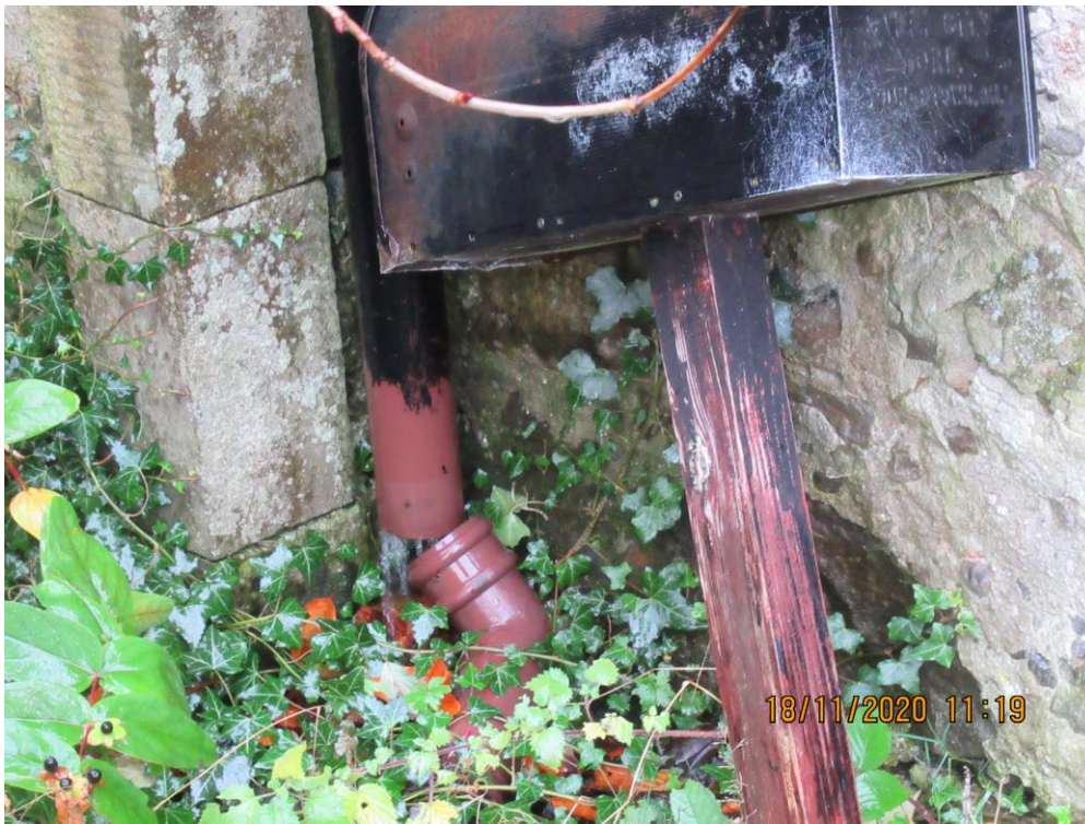
This photo is of the same down pipe at the lower section. It shows the pipe being disconnected and flowing directly onto the ground.
