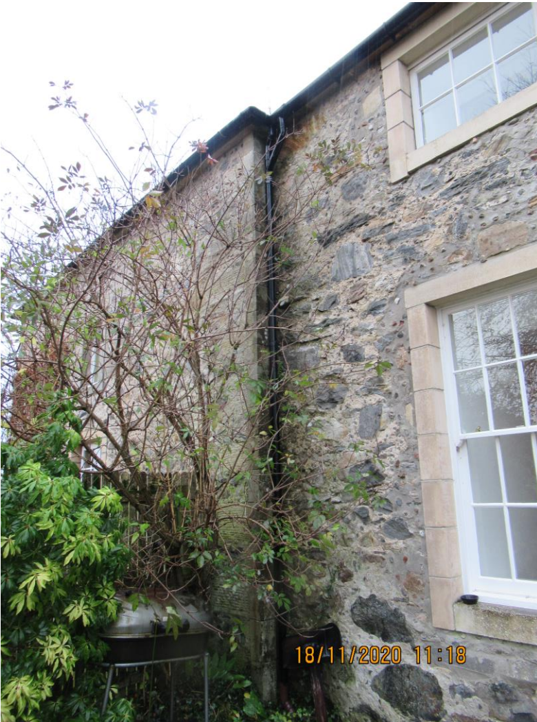
The down pipe to the left of the front door was overflowing from the top and you will notice the beginning of algae staining on the masonry in behind the pipe. Possibly just needing to be cleaned out.
