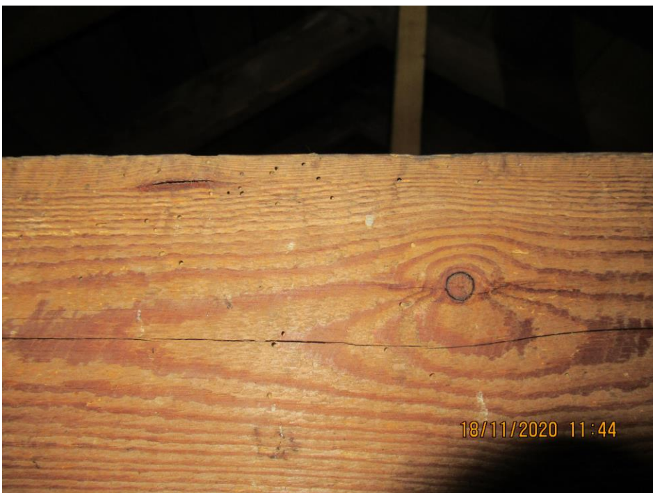
This photo shows a roof timber where the woodworm infestations are “inactive”. It is highly probable that woodworm treatments were carried out during the renovation of the roof.
