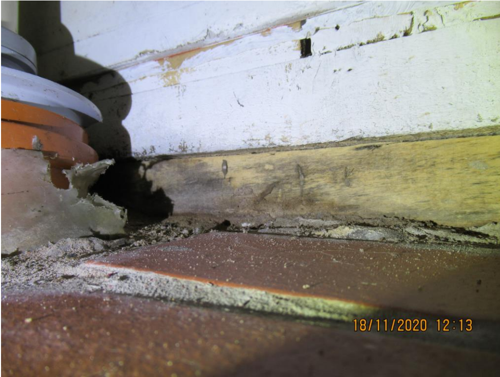
Slight surface decay to the lower grounding timber.
