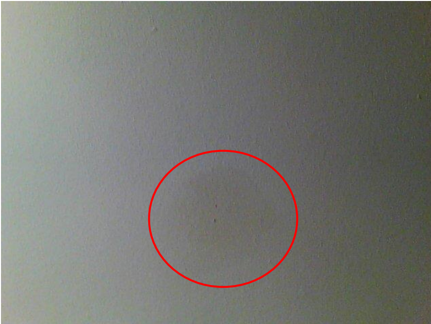
Historic damp stain in the ceiling
