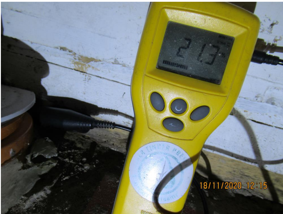
Moisture readings of the isolated area reads 21.3%, which is still considered as "slight". If desired and as a precautionary measure, the affected area can be chiselled out and a preservative brush applied.
