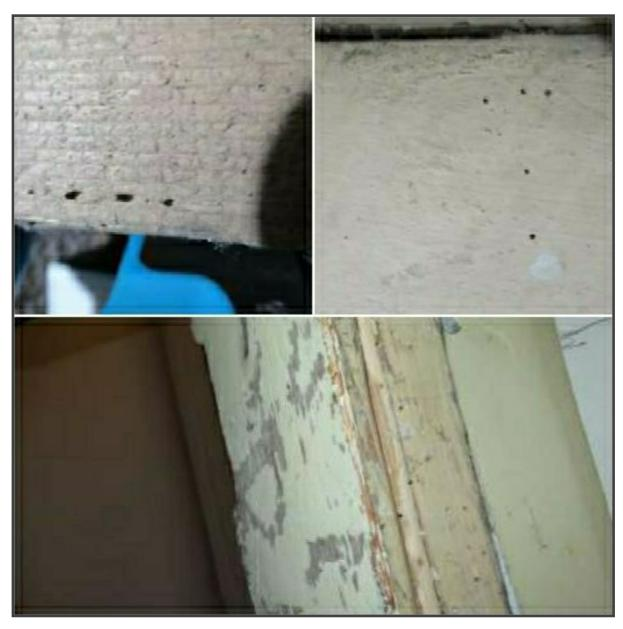
At the time of our survey old activity by the common furniture beetle (Anobium punctatum) was evident to the floor and door frame timbers within the under stair cupboard area. No active woodworm infestation was noted and no treatment is required.
