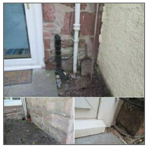
External ground level was previously in area's in relation to internal floor level (this has recently been corrected by the client).
